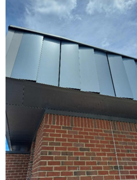
Aluminum fascia panels
