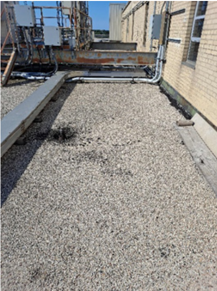
Existing roof - replace
