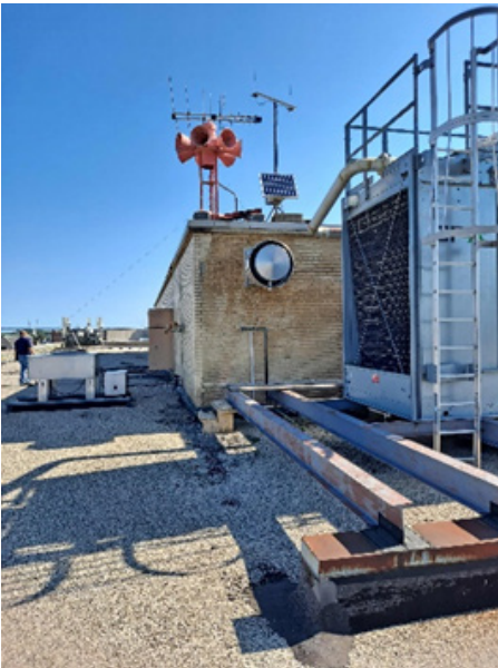
Existing roof - replace
