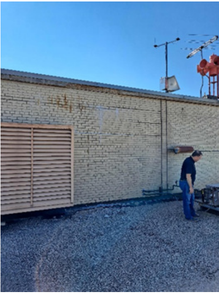
Mechanical penthouse - tuck pointing
