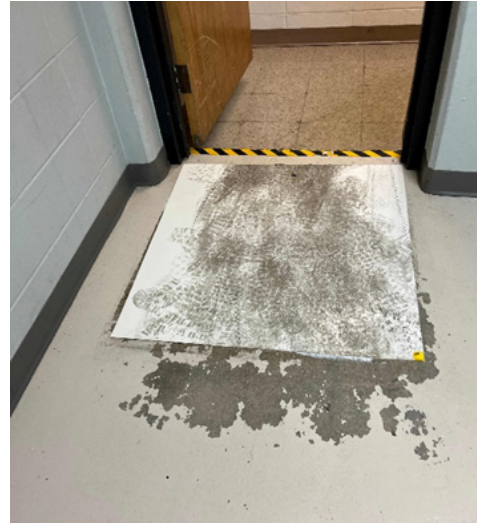
Chipped paint at shooting gallery entry
