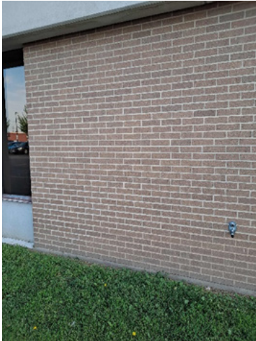
Brick in good condition
