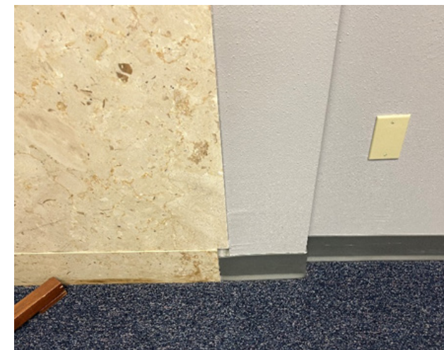
Fill gap in wall
