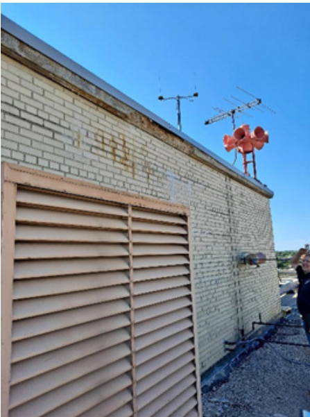
Penthouse pre-cast coping replacement
