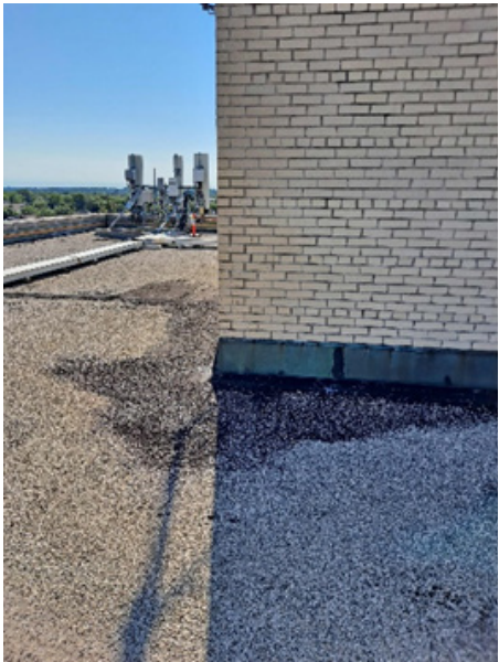
Mechanical penthouse - tuck pointing
