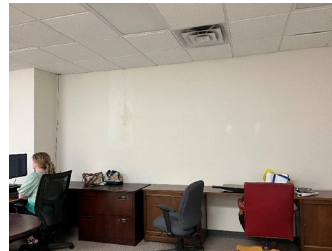
Visible wall patches
