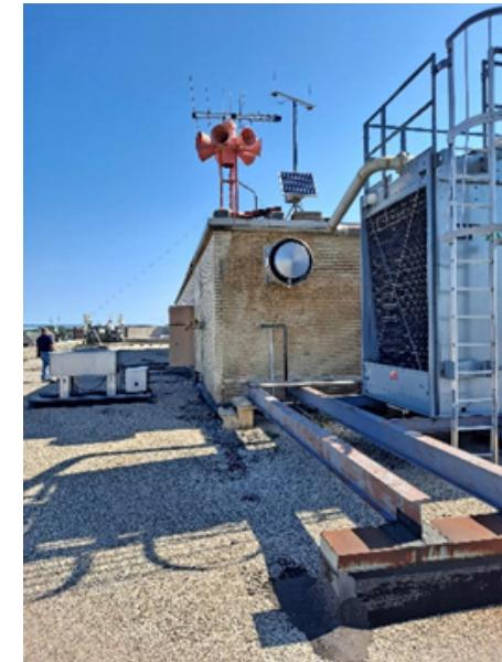
Existing roof - replace
