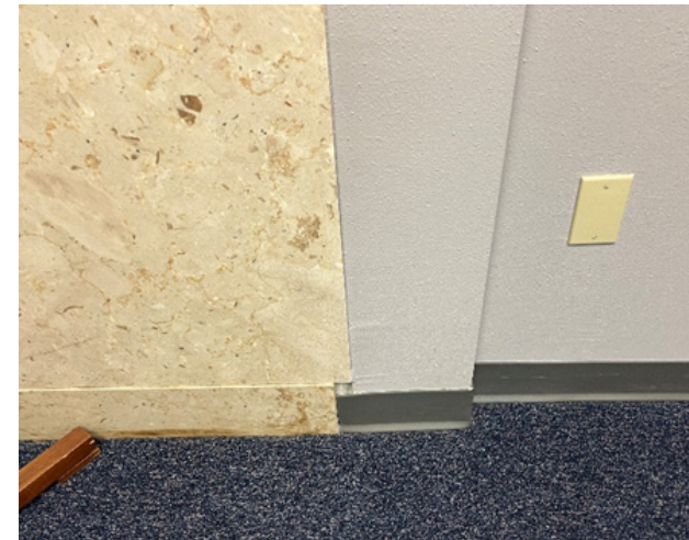
Fill gap in wall
