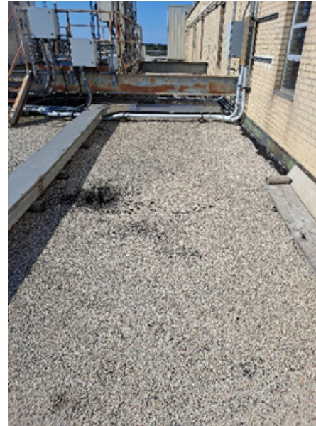
Existing roof - replace
