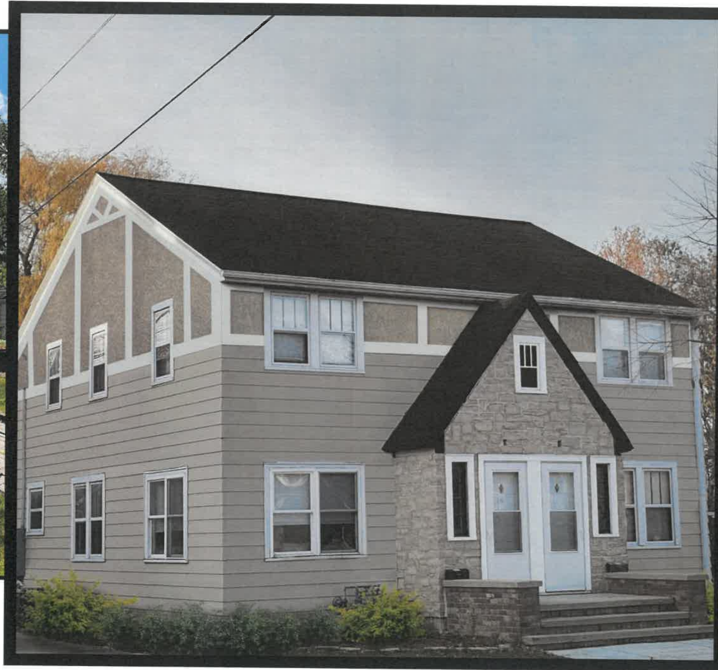
IN PROCESS - STONE & SIDING
