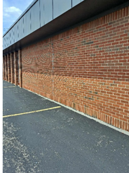
Exterior brick in good condition
