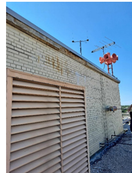
Penthouse pre-cast coping replacement
