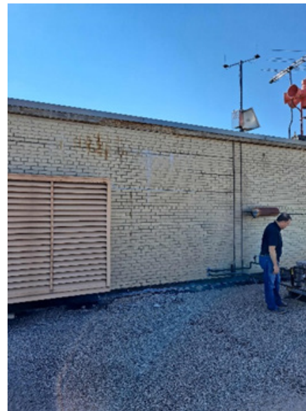
Mechanical penthouse - tuck pointing
