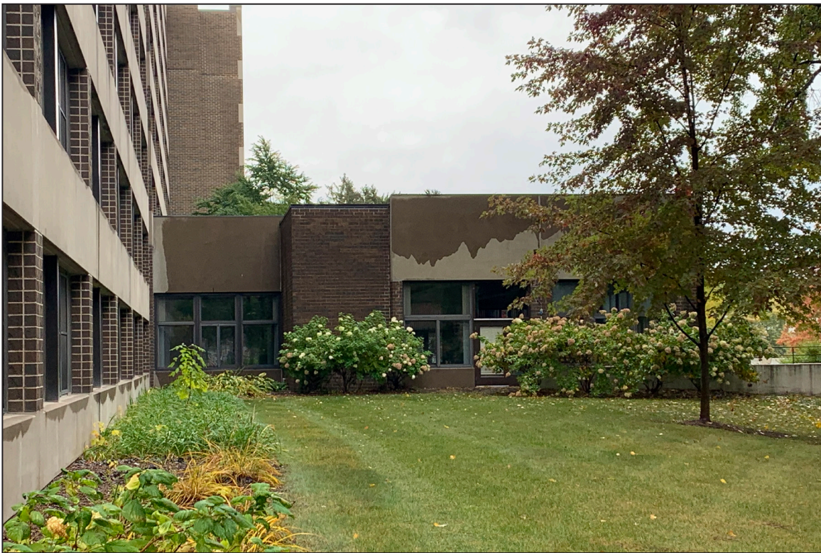
18. Community Center, South Elevation, looking north.
