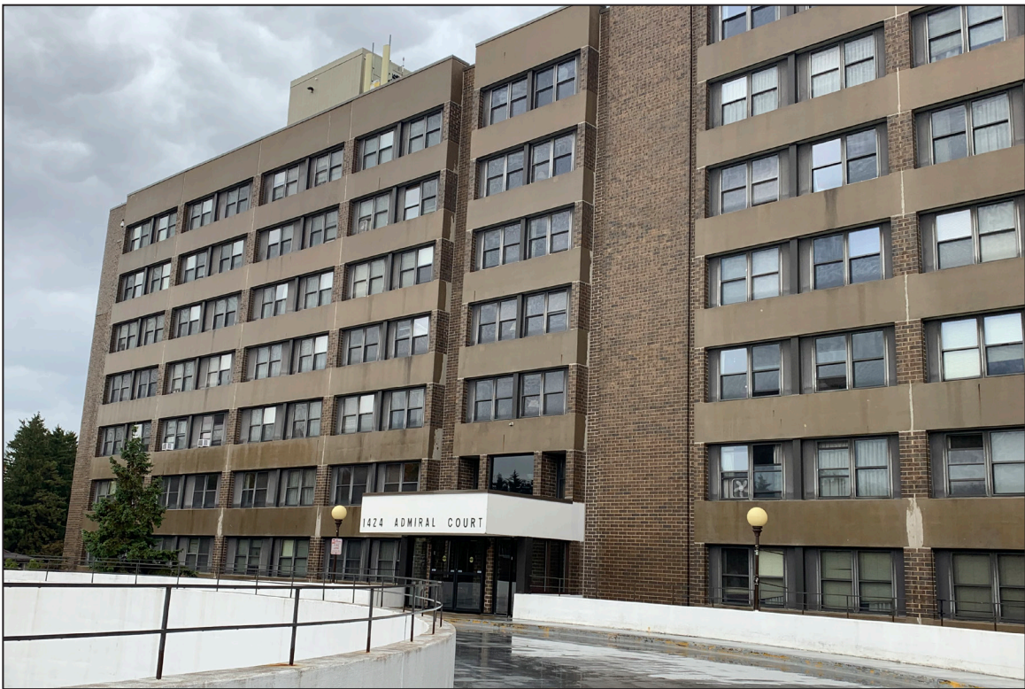
2. West Elevation, looking northeast.
