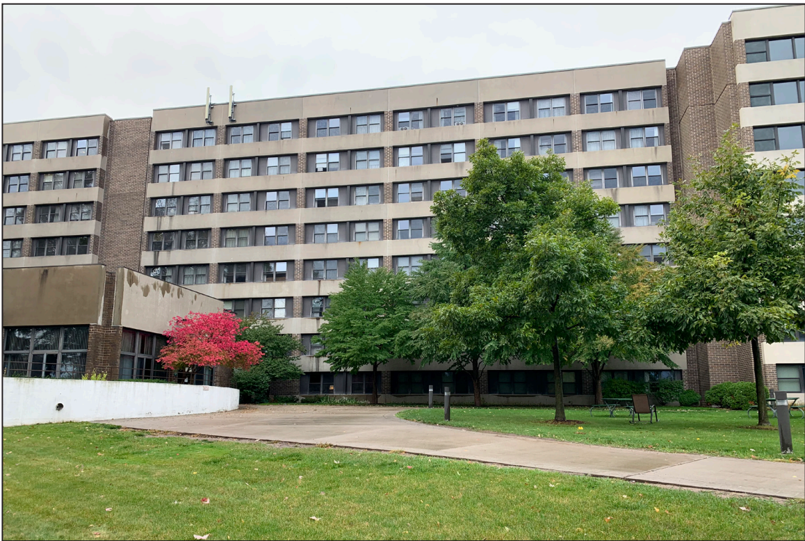
14. East Elevation, looking west.
