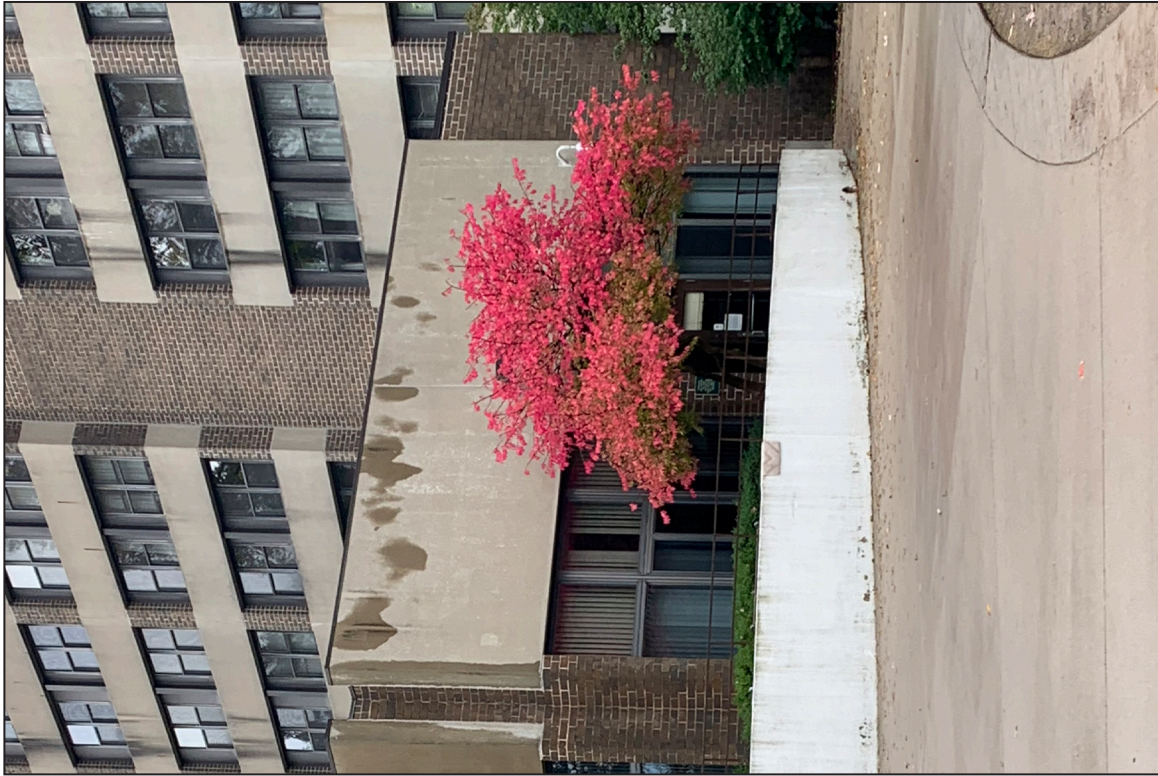
15. East Elevation, looking southwest.
