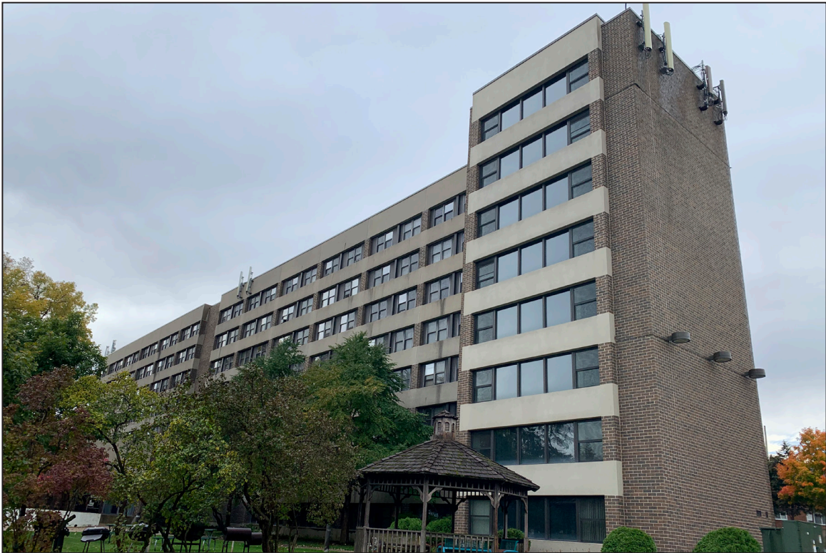
12. North and East Elevations, looking southwest.
