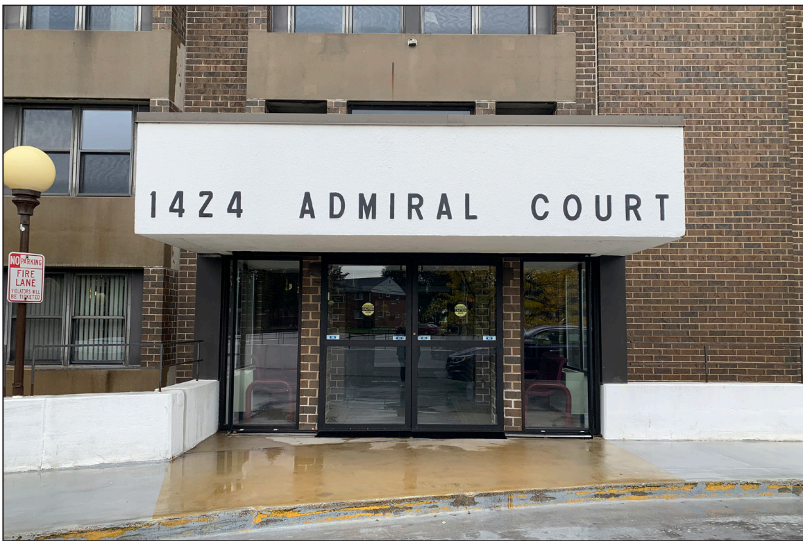
6. West Elevation, looking east at entrance.
