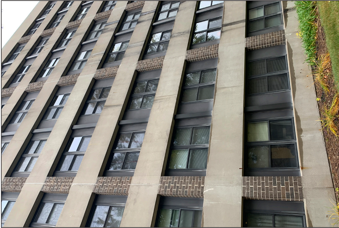
17. East Elevation, looking west.
