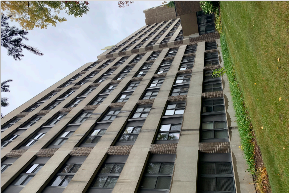
16. East Elevation, looking northwest.
