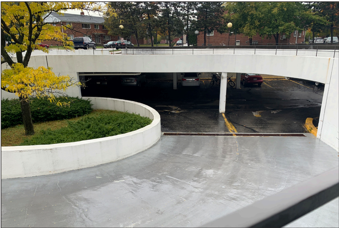
22. Garage, looking northwest at entrance.
