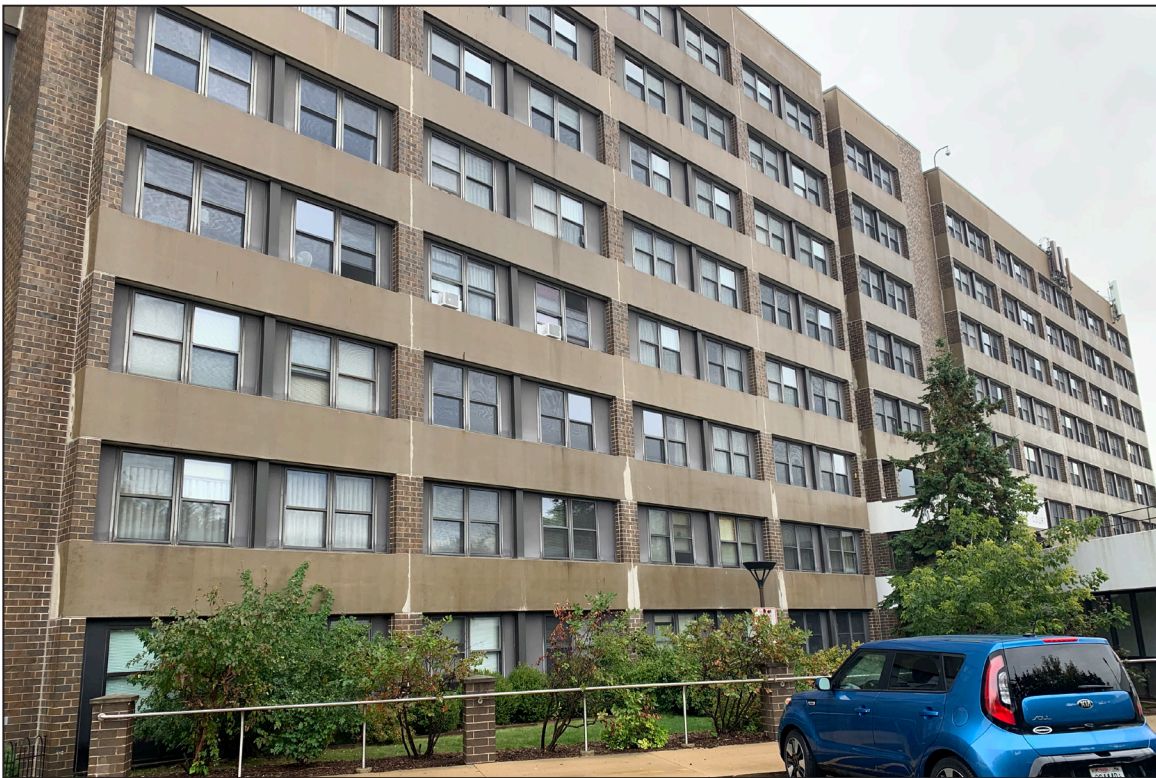
8. West Elevation, looking southeast.
