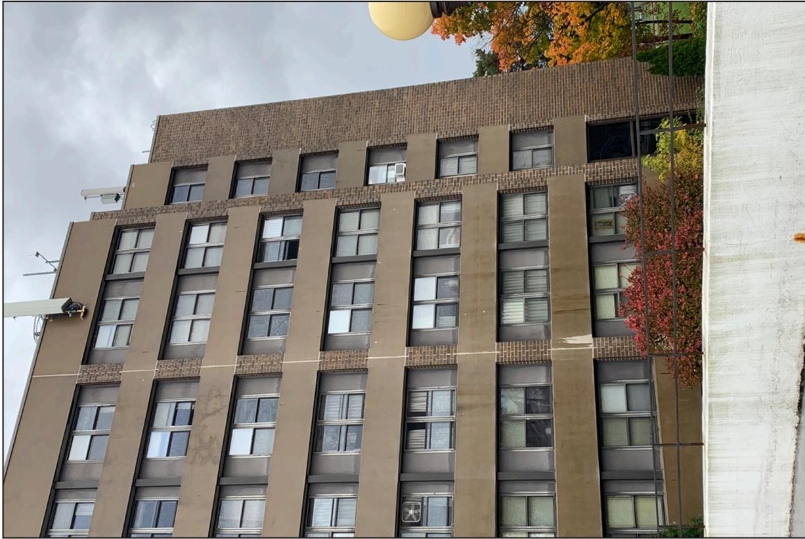
3. West Elevation, looking southeast.
