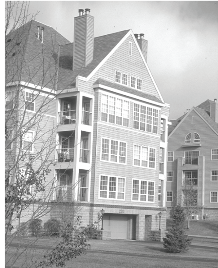
Example of senior multifamily apartments.
