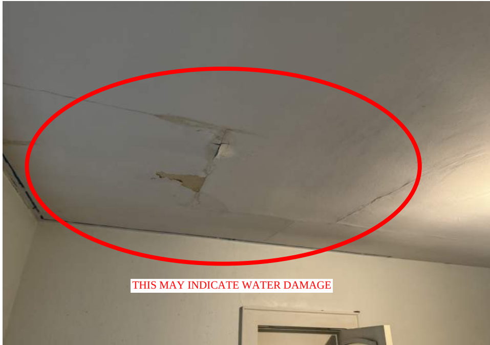
DAMAGE AT TUB
