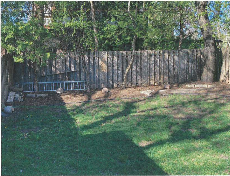
EXISTING FENCE AT NORTH LOT LINE
