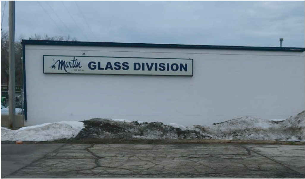
Remove Existing Wall Cabinet Sign
