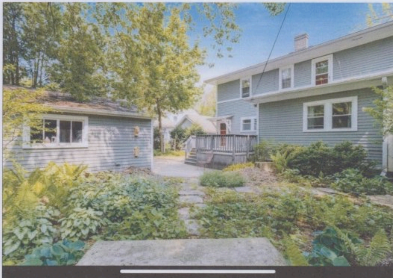
812 Cass St. (Rear View) Additional photo showing 1 st floor addition
