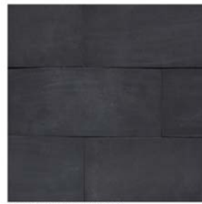
EXTERIOR STONE MASONRY #3 (Sill Condition)
