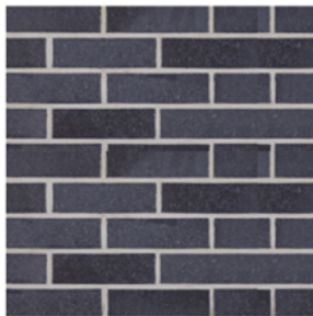
EXTERIOR BRICK MASONRY #2
