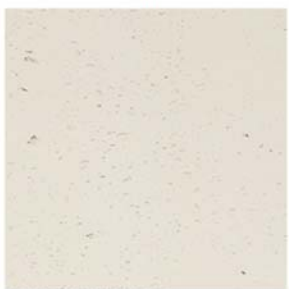
EXTERIOR STONE MASONRY #1 (Pedestal of Columns condition)
