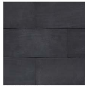
EXTERIOR STONE MASONRY #3 (Sill Condition)
