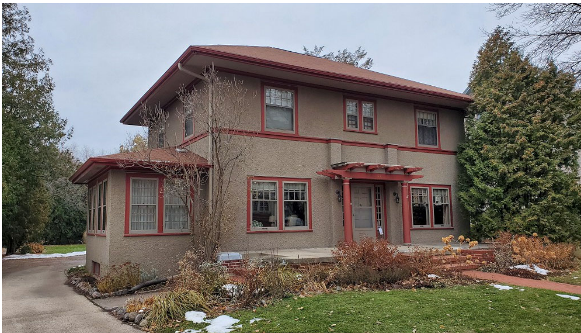
View from adjacent sidewalk, 2019
