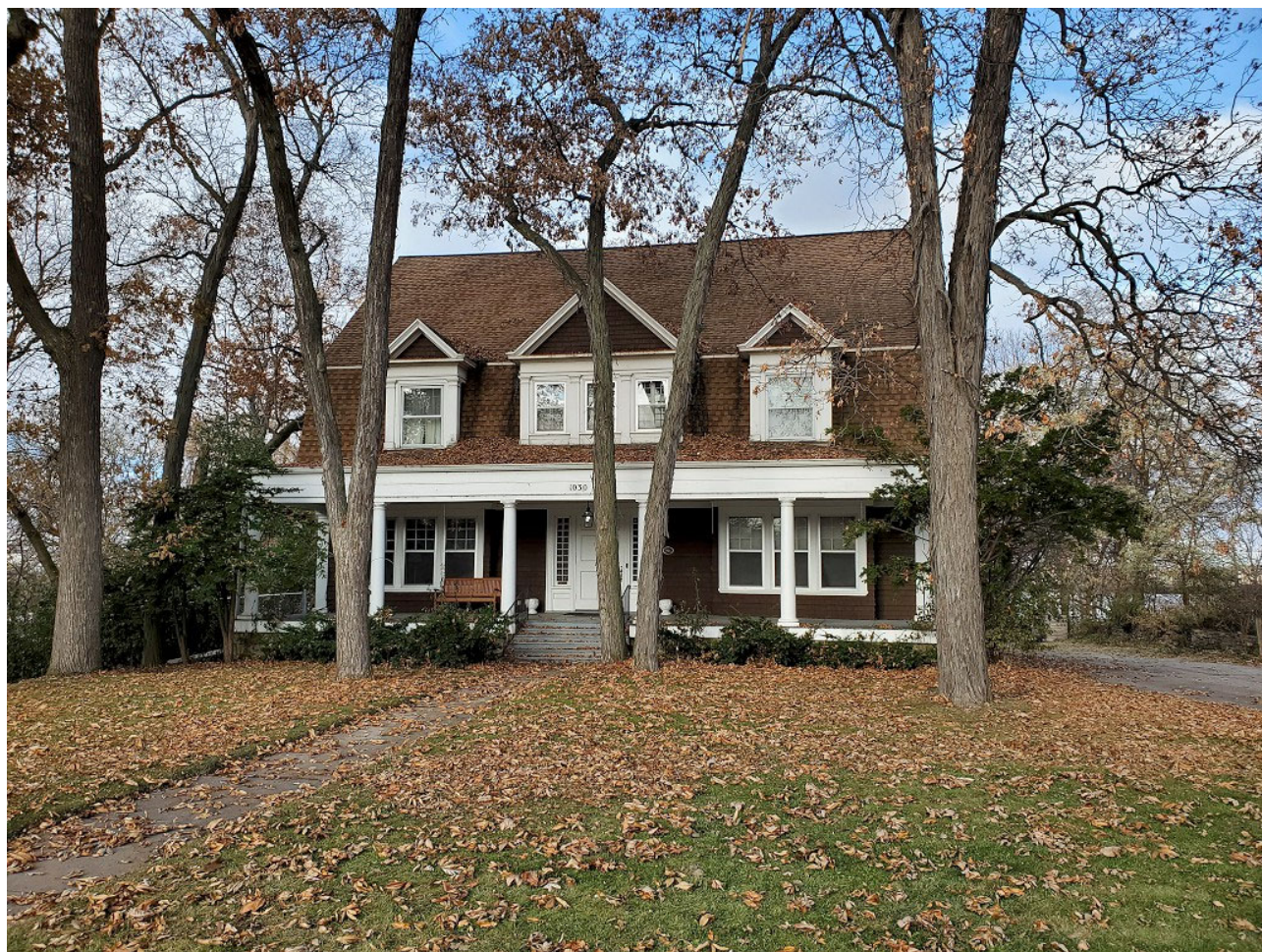
View from adjacent sidewalk, 2019
