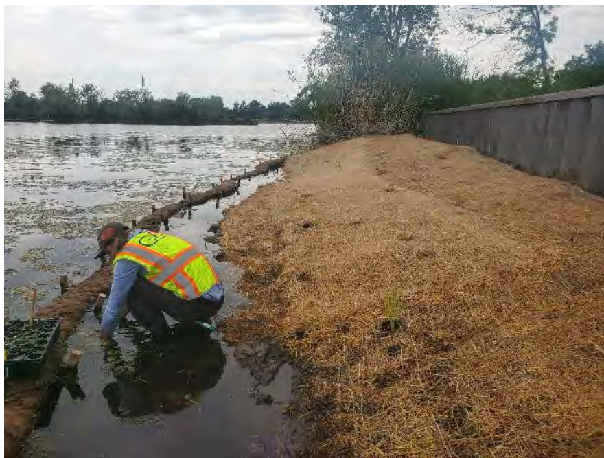
Figure 10. Restoration site where submergent marsh plugs are planted underwater. Note the plugs planted through the erosion control blanket to the right of the GEI staff member.
