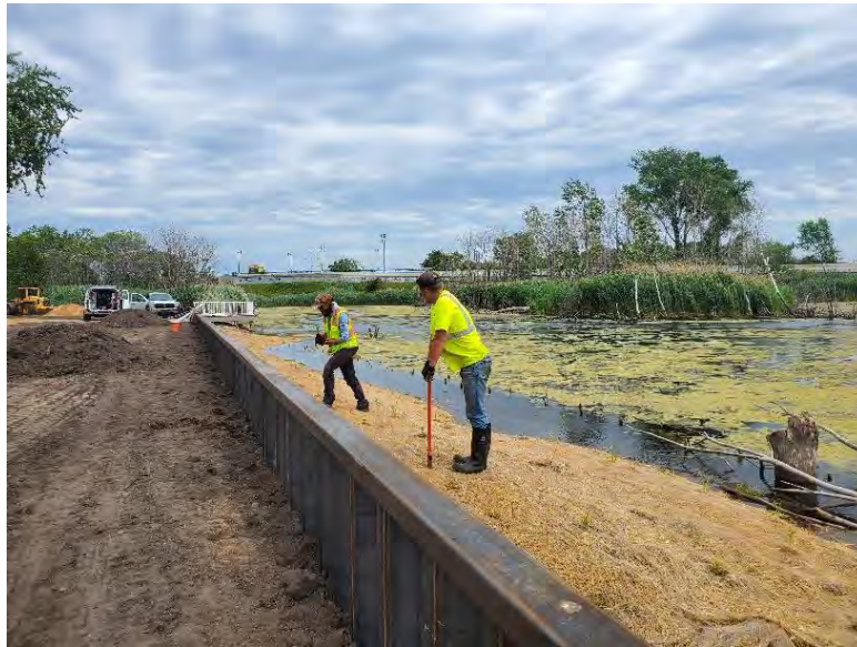
Figure 11. Project site restored by GEI in Menominee, Michigan showing erosion control blanket placed and plugs planted through openings in blanket using tree bars.
