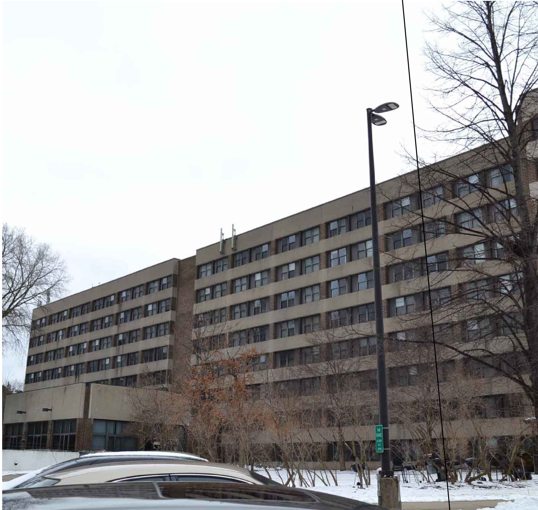
1 OVERALL BUILDING PHOTO
