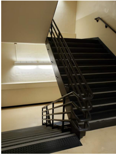
Room 300A, typical stair assembly.
