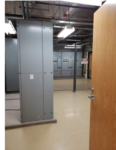
Room 203, looking east.
