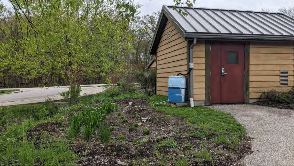
Rain barrel to rain garden
