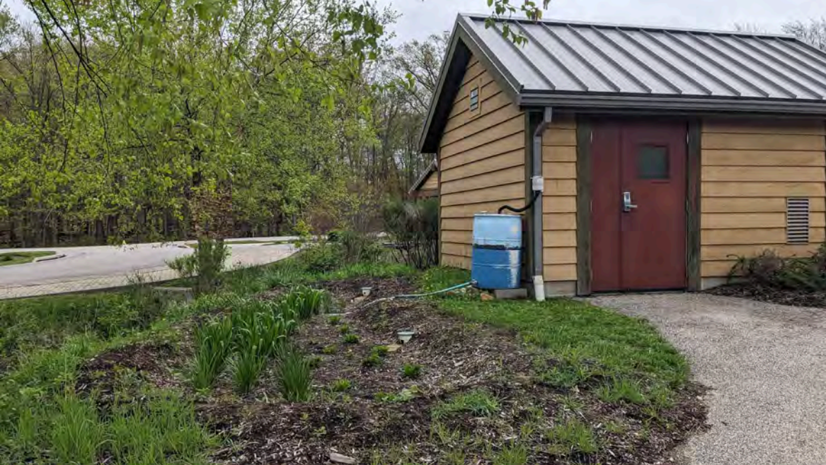
Rain barrel to rain garden
