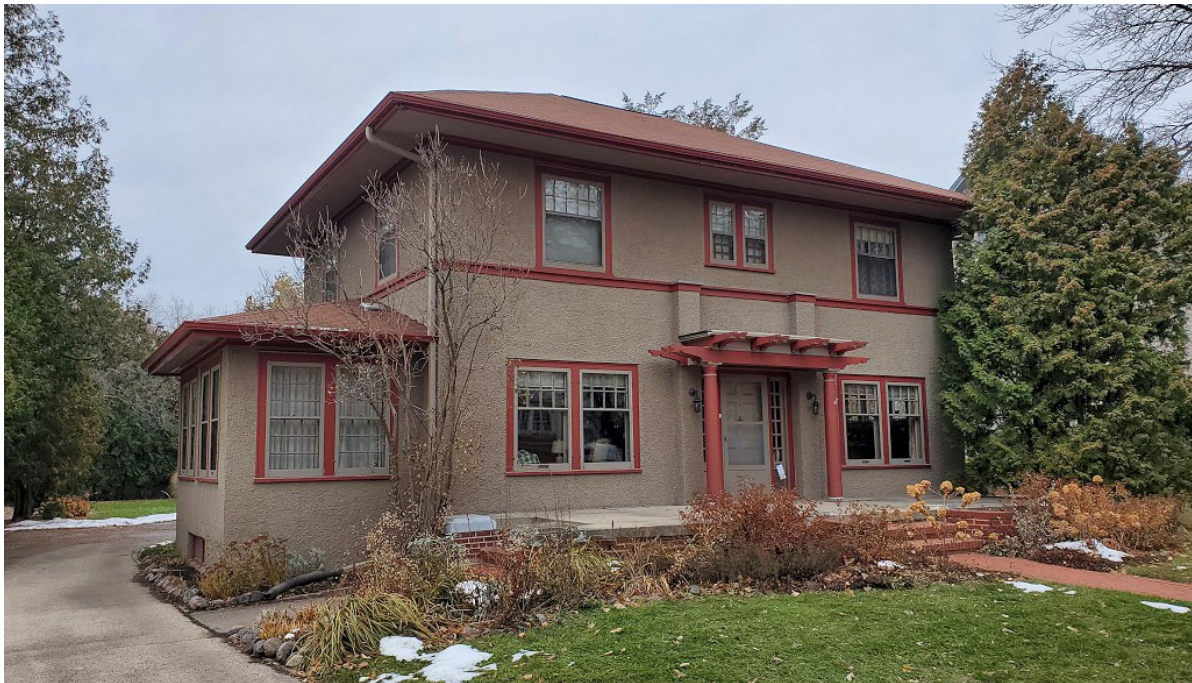
View from adjacent sidewalk, 2019
