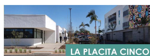
A strip mall transformed into workforce housing.
