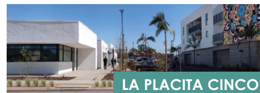
A strip mall transformed into workforce housing.
