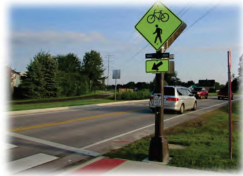
Rectangular Rapid Flashing Beacon (RRFB)
