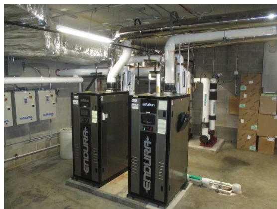
Typical Interior View
