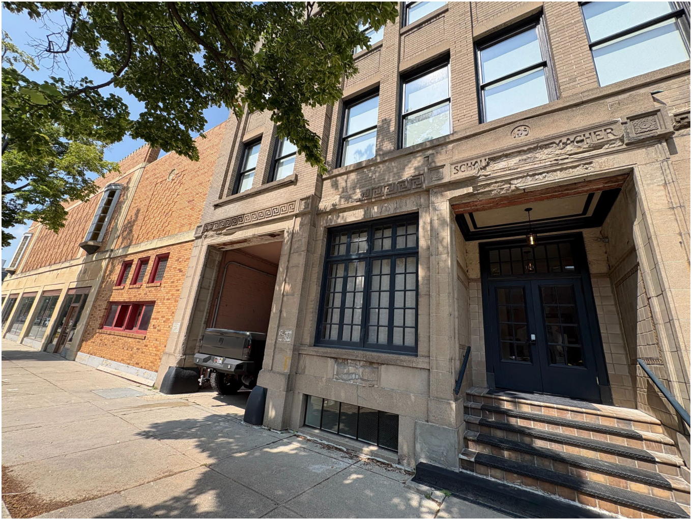
Existing facade - oblique view showing the building and adjacent streetscape.
