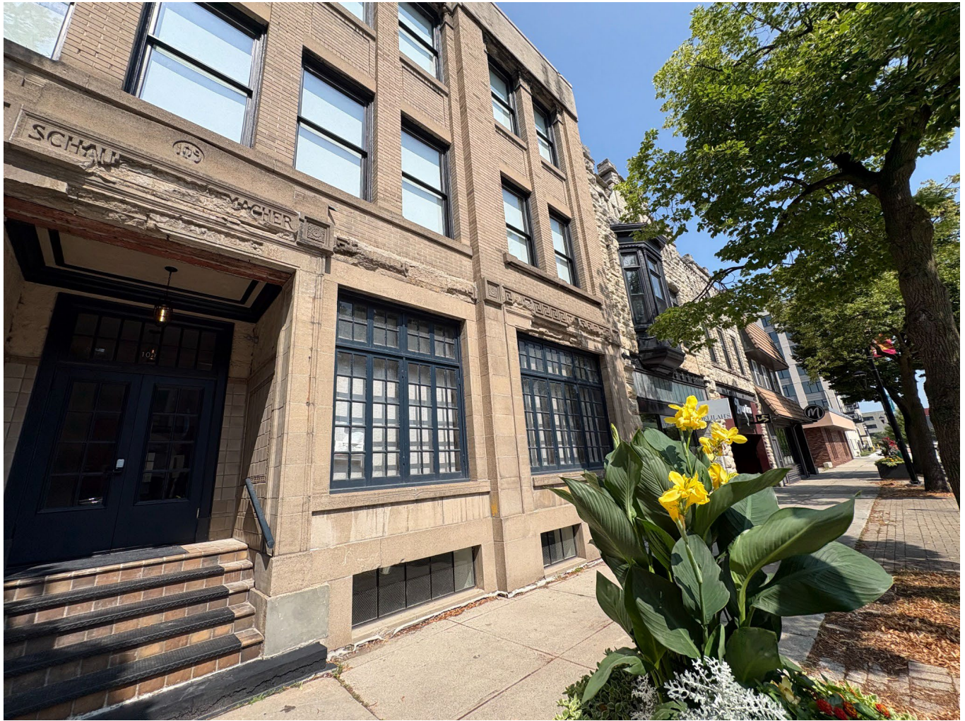
Existing facade - oblique streetscape view looking along N. Adams Street.
